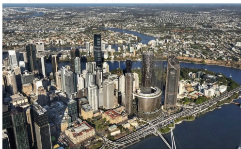
Australian Real Estate Property
